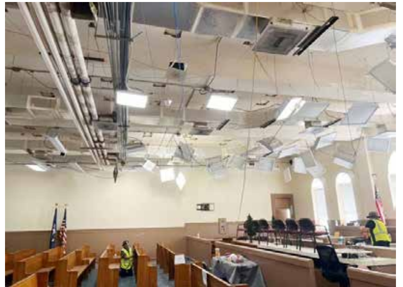
A courtroom under renovation in the Pointe Coupee Parish Courthouse.
