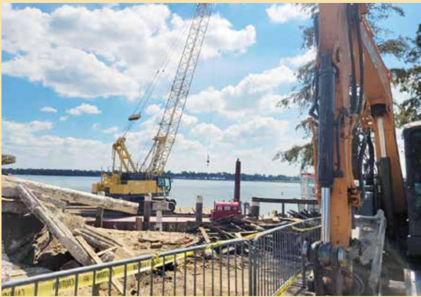
Repair of the bulkhead in downtown New Roads.
